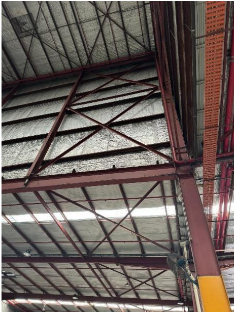
I12-04 Source p.12 middle-right Stacked upper braces, IF1 junction, adjoining lower roof and attached service runs.
