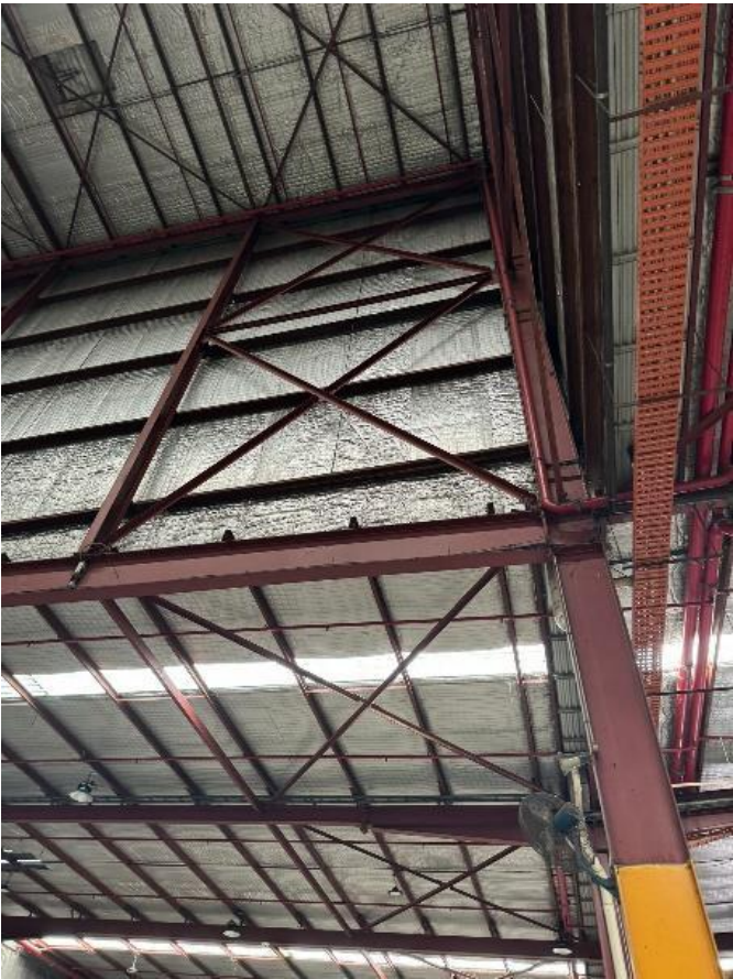
I12-04 | source p.12 middle-right Upper braced wall above lower roof; horizontal interface framing and attached service routes.
