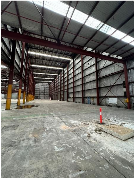
I10-04 Source p.10 middle-right Full-height enclosure, horizontal girts, rooflights and bracing before strip-out.
