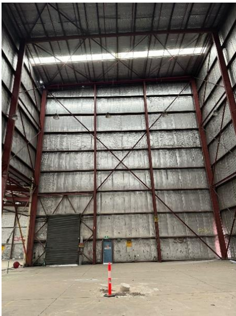
I14-06 Source p.14 bottom-right End posts, diagonal arrangement, girts, door and rooflight strip; correlate end orientation.
