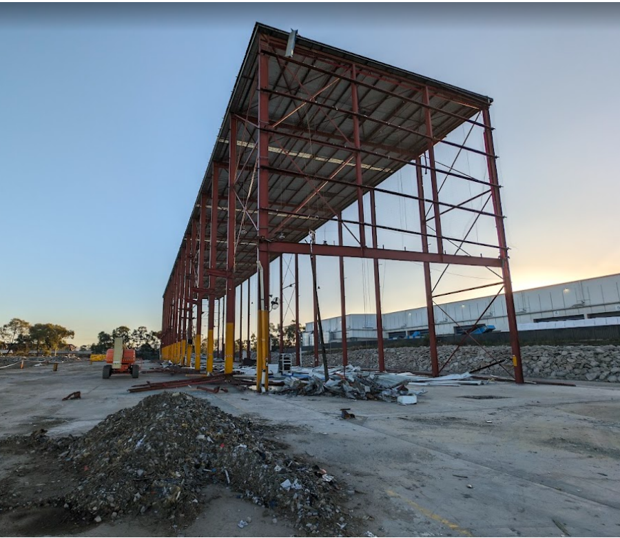
P04 - STRIPPED WALLS / RETAINED ROOF
