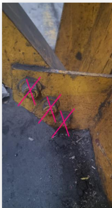
Figure 10: Cutting specifications for column weakening
