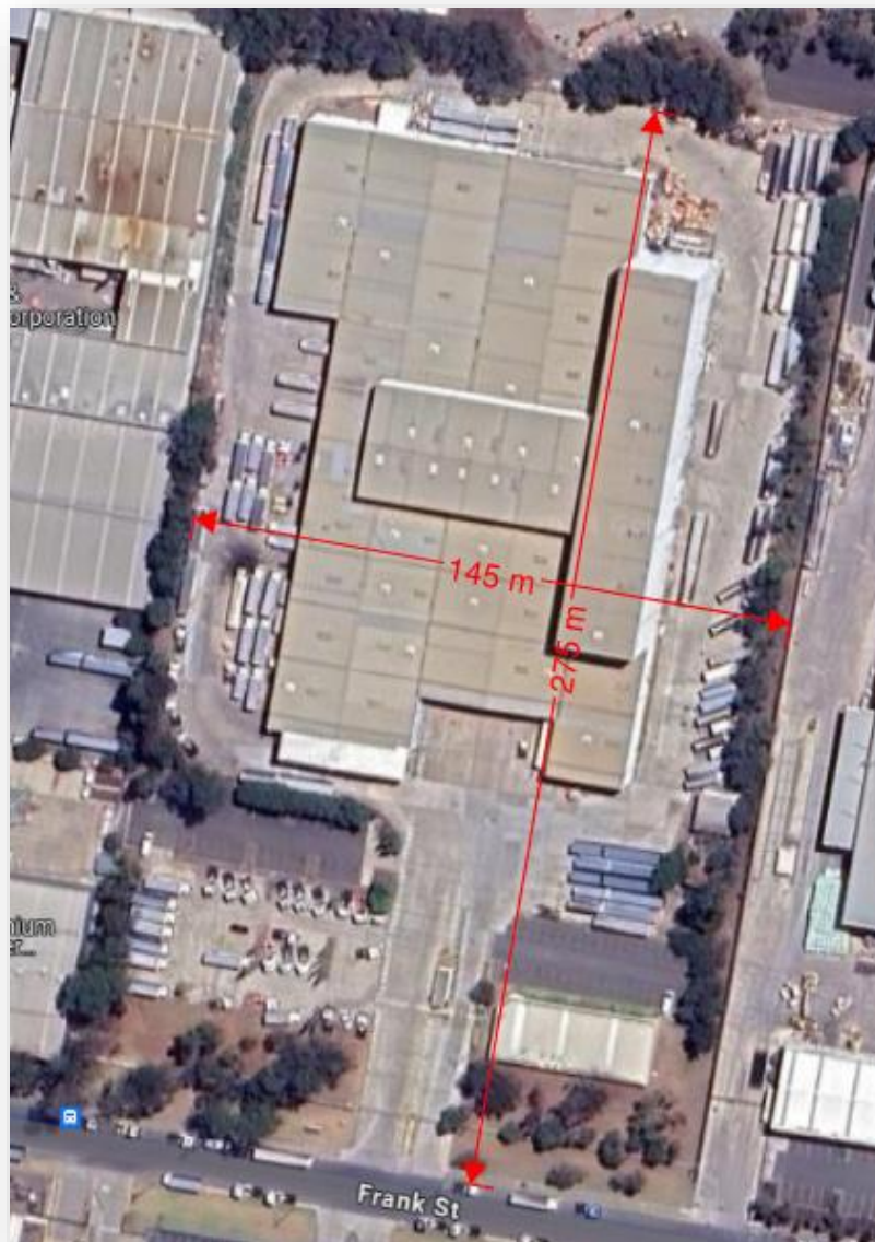
Figure 1: Aerial view of 27 Frank Street, Wetherill Park, NSW, 2164
